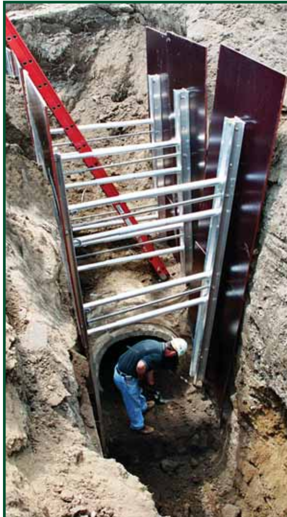
12 ft. Hi-Clearance Shores, 16 ft. stacked FinForm, Lifting Sling, and Pump Can
