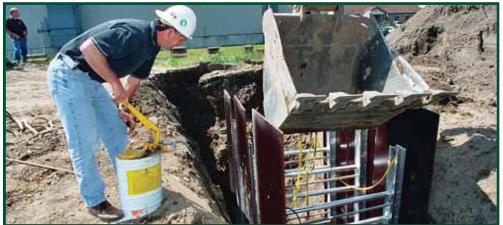
12 ft. Hi-Clearance Shores, 16 ft. stacked FinForm, Lifting Sling, and Pump Can
