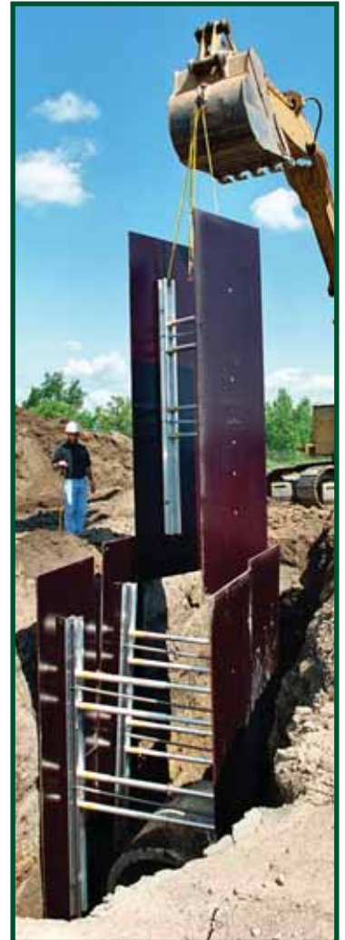
12 ft. Hi-Clearance Shores, 16 ft. stacked FinForm, Lifting Sling, and Pump Can
